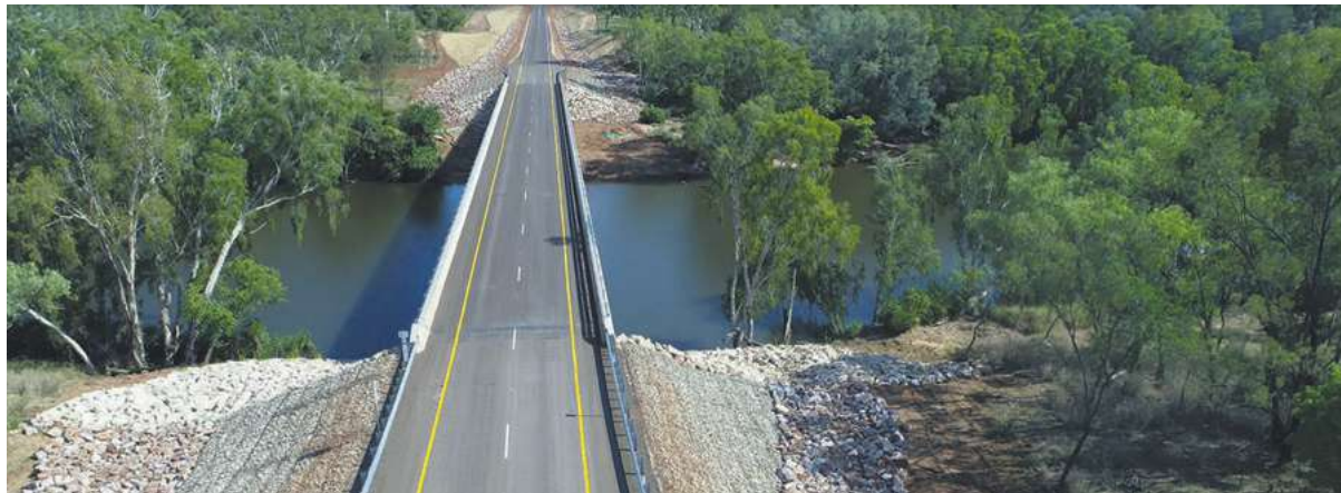
Yurhunj Bridge over Roper River
